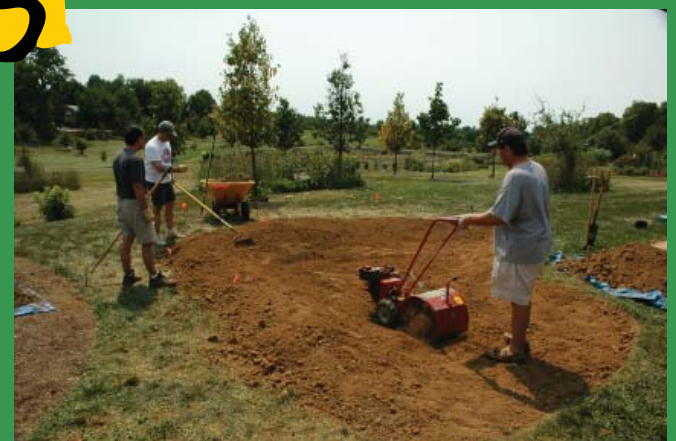
Dig, add soil modifications, mix soil & level*
